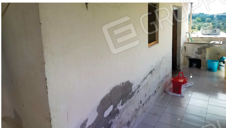
(Foto n.9_ balcone-veranda piano secondo)
