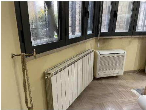
Foto 11: muffe in camera matrimoniale
